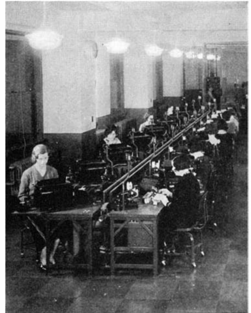
Special wires lead from the room at the right to 40 important offices throughout the country where cable traffic is collected. These wires connect to printing telegraph machines from which the messages go on their way to various foreign lands
