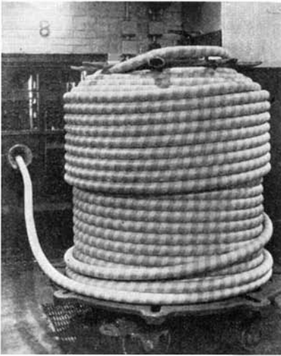
The cable after manufacture is wound with paper and is given a thorough drying in vacuum driers that discharge the "bone dry" cable into a low humidity storage room when it goes directly to the lead sheathing presses as it is needed. The protective covering of lead is the last process in cable manufacture
