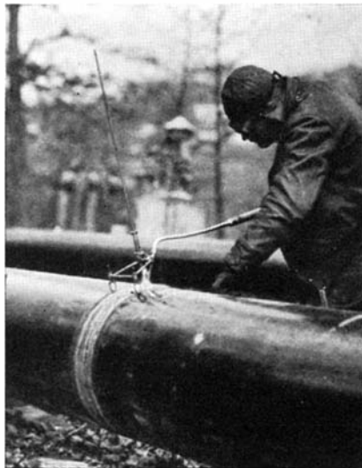
The new oxy-acetylene welding torch, in use, is almost automatic
