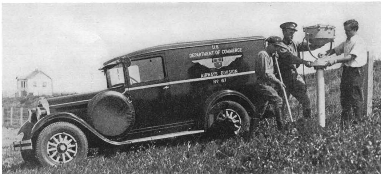
Installing a ceiling light on an intermediate landing field. This light will be used in connection with the clinometer shown in the photograph at the top of this page, and its rays can "spot" clouds 7000 feet high. Airway keeper's home is at left
