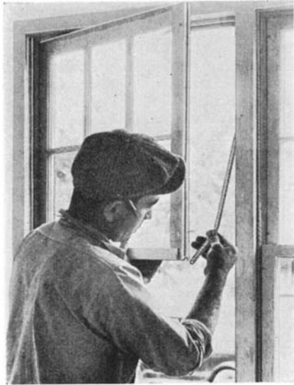
Strong tension springs used to replace the usual window sash weights
