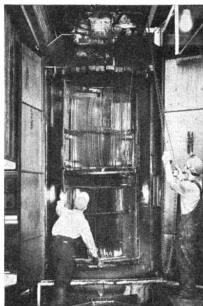
Racks of preliminary pressed Duplate being lowered into autoclave
