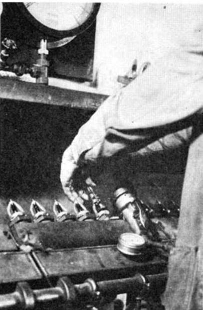
Pressure testing and adjusting bulb to insure proper tightness of seat
