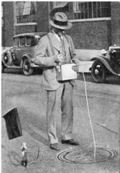
Explosive gas tester in use
