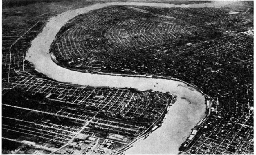
Where more than 100,000 quartz bulb sprinklers have been installed in the docks on the right hand side of the Mississippi River in the city of New Orleans
