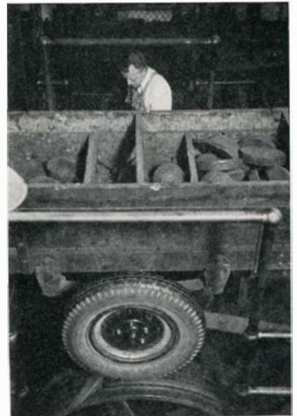
At the left is shown a Jumbo tire in the "pile-driver" ready for the bruise-break test. Dropped repeatedly onto the anvil as shown above, and other anvils of various shapes, the tire sustains many kinds of fabric breaks and tread bruises
