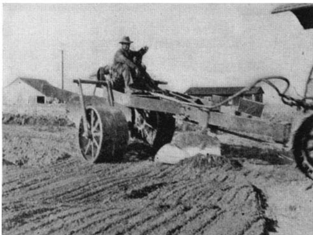
The huge plow which was built especially for the job of "renewing" the fertility of a sand-covered western valley
