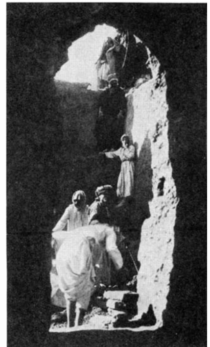
Working at low level, baskets containing earth are passed by hand
