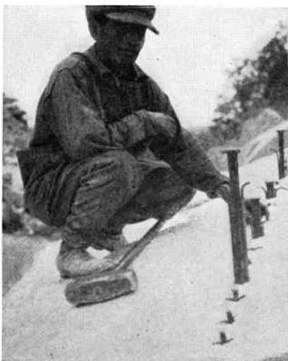
Left: Bars and wedges, inserted in holes, start a crack on a bench and will finally break off a huge block
