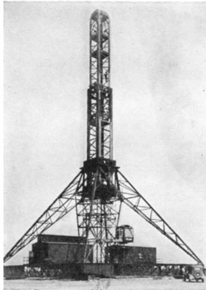
The new telescopic airship mooring mast in its high extended position
