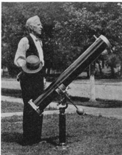
Henry C. Kawecki, Massachusetts Institute of Technology Dormitories, Cambridge, is a student of electro-chemical engineering, but in summer vacation he made a portable reflecting telescope. "Little trouble was encountered," he says. The telescope has a worm-and-gear slow motion, also setting circles
