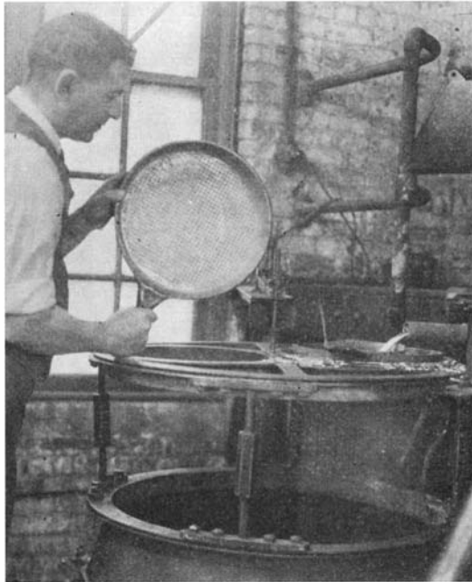
The melted lead or alloy passes through the hundreds of holes in an iron sieve, and falls in globules to the tank of water 120 feet below
