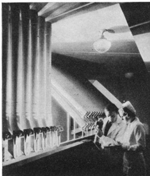
A pneumatic tube system transports medicines as well as letters, records and so on
