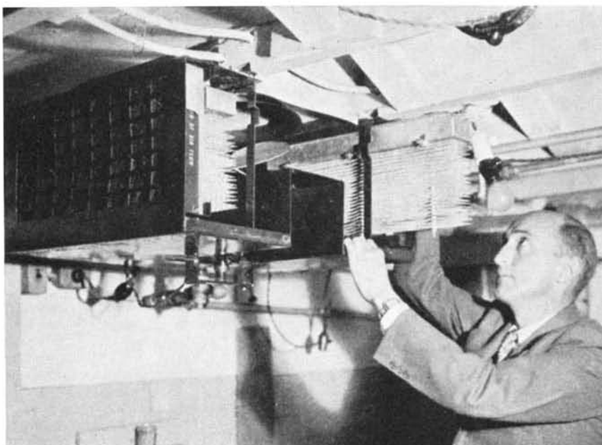
An air humidifier and filter being installed in a private home
