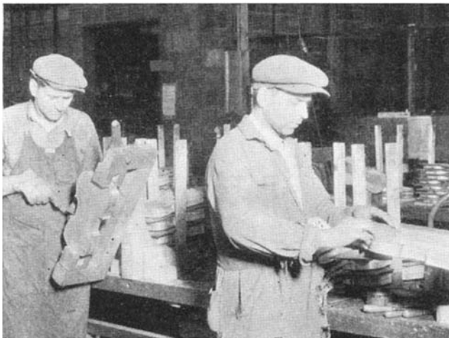
Filing and otherwise smoothing the panels in order to remove dead metal accumulated during welding process
