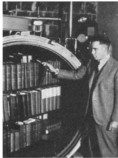
Above: Top indicator points to a beetle; others to bookworms at work. Right: Vacuum fumigator used in war against destructive bookworms
