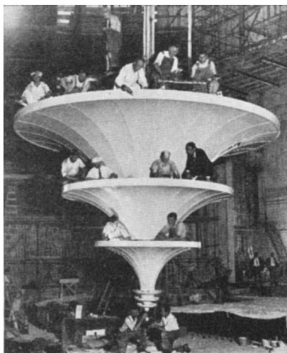
World's largest chandelier being installed at Rockefeller Center, New York City. Three hundred flood lamps consuming 104,000 watts will require a special ventilating system to carry off the heat
