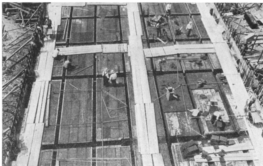
Heavy corkboard insulation is used in the new M.I.T. laboratory
