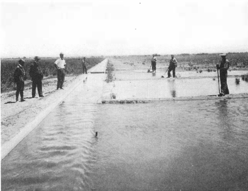
Irrigating a large field, broken into sections by means of miniature diversion dikes, from a concrete-lined ditch on the Salt River Project in Arizona
