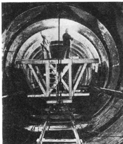
Laying caulking welds in assembled sections of new water tunnel liner
