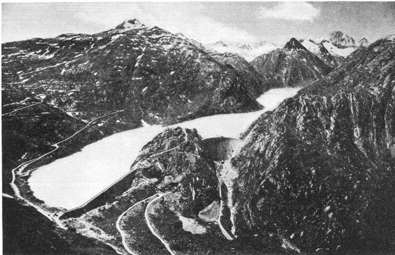
Grimsel Lake and the two dams which create it; a hospice on the peak between the dams; and a motor road
