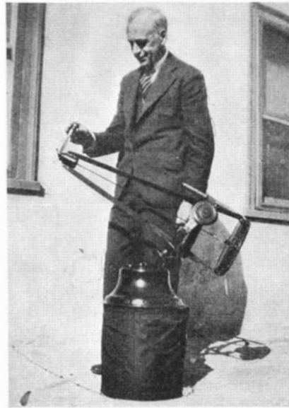
Below: Kenneth N. Reed, 268½ North Los Robles Ave., Pasadena, California and an 84-pound portable nine-inch telescope made at the very low cost of $4.88. Two unique pipe braces take the place of the tube
