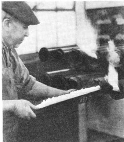
Painless extraction with gas. Tungsten oxide is inserted into the flaming trough of a hydrogen furnace at the Westinghouse Lamp Company. Three hours of this and all moisture has been extracted, leaving powdered metal tungsten. This powder is placed in huge presses and pressed into solid metal for drawing into lamp filaments
