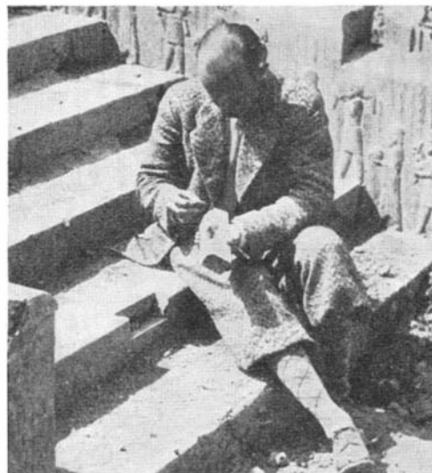
Right: The step was repaired by a carved piece set with lead. A defect in the figures was remedied by carved lead. Below: Small stairway with relief sculptures in stone
