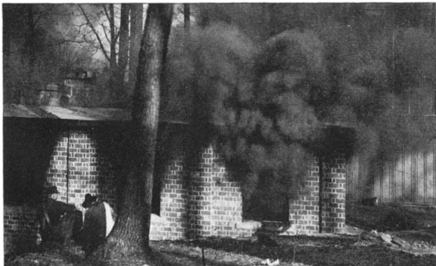
When the Bureau of Standards wants to know facts concerning the duration and intensity of fires, they do not theorize, but instead simply start a fire in this building, after furnishing it to simulate any desired occupancy. The temperatures are then measured at many points within the house by thermocouples
