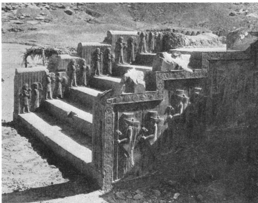
Right: The step was repaired by a carved piece set with lead. A defect in the figures was remedied by carved lead. Below: Small stairway with relief sculptures in stone
