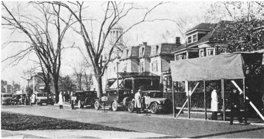
A typical Safety Lane with headlight-testing section at the right
