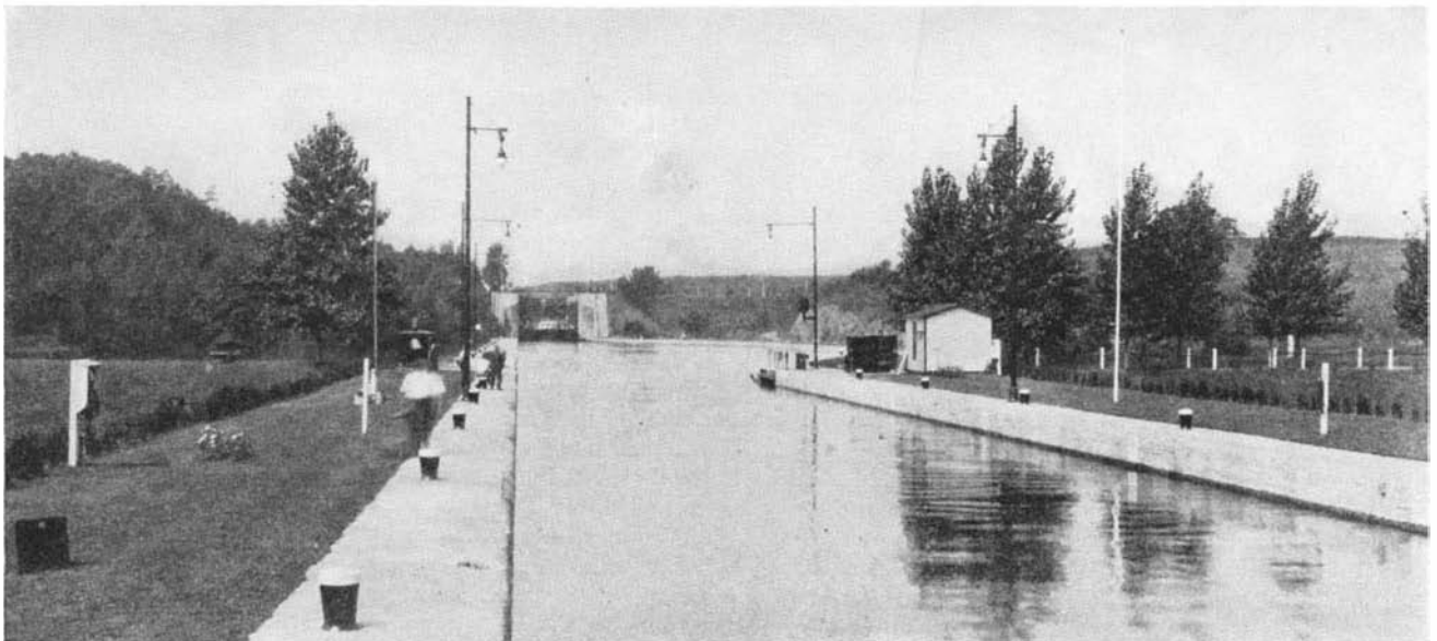
View of Waterford flight of locks on the Erie Canal, showing a motorship just leaving the distant lock 4 and approaching lock 3 in the foreground. There are five locks within two miles in this group which raise or lower a vessel some 169 feet
