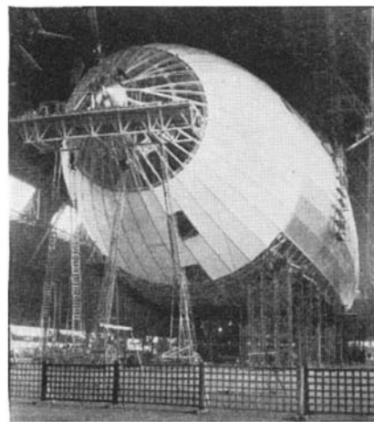
Applying outer cover to the Macon
