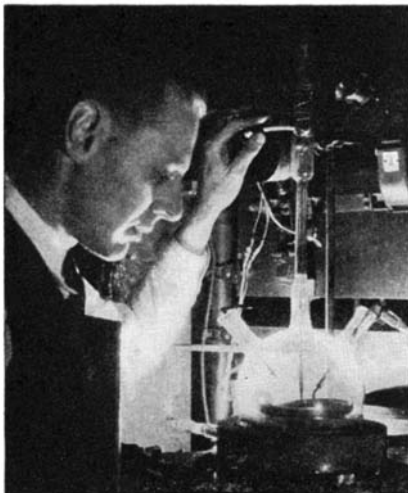
The "ignitron," in which a tiny current applied to a pencil lead controls enormously high currents
