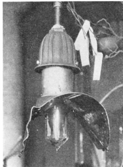
Close-up of sodium vapor lamp with its curiously designed reflector
