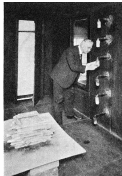
Outside the fire test room, showing connections for sampling the gases
