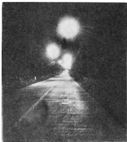
Experimental installation of new sodium vapor lamps on a highway
