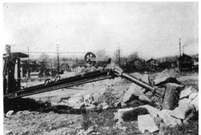
Two views of the traveling power hammer, described above, in use for breaking rocks
