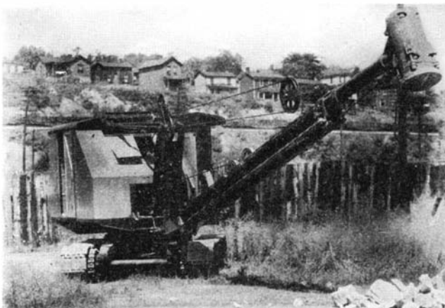
Two views of the traveling power hammer, described above, in use for breaking rocks
