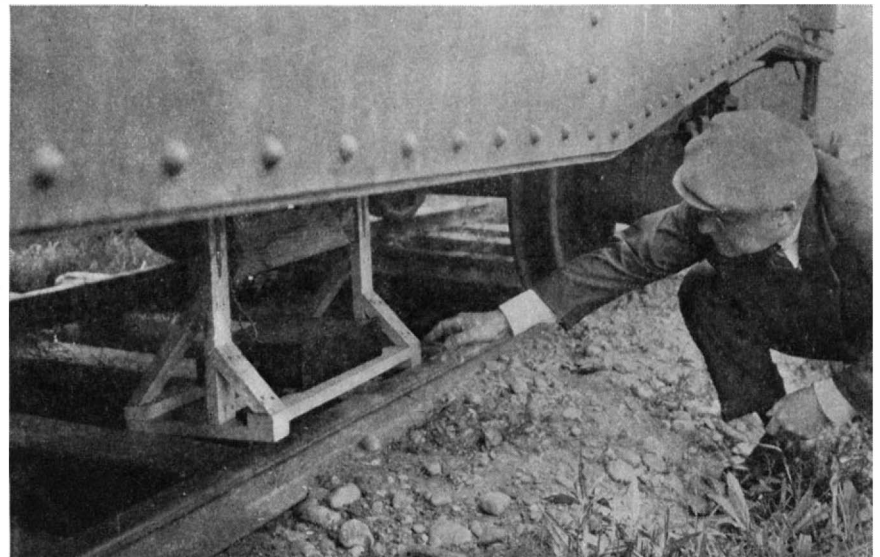
The inductor coils, used in connection with the freight train communication system described above, are hung on special brackets just above the rails
