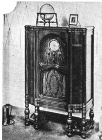
A circular tuning dial with four different scales is a feature of this particular all-wave receiver
