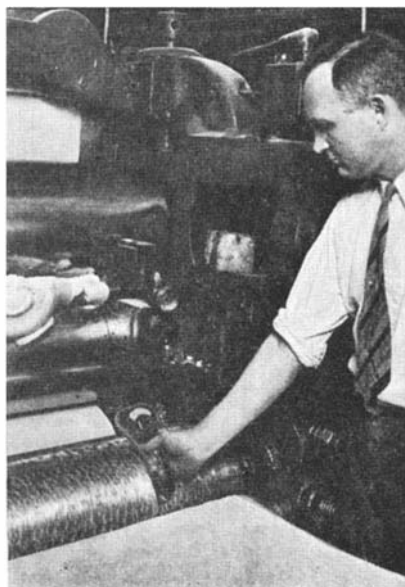
A portable temperature indicator that will work on curved surfaces
