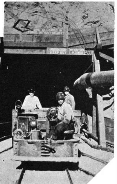
Below: A storage-battery locomotive. Note steel helmets on workers to prevent head injuries
