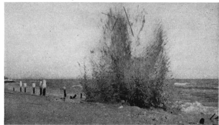
One charge at the middle of the line was primed with a cap but detonation set off the five charges on each side—eleven with one "sh"
