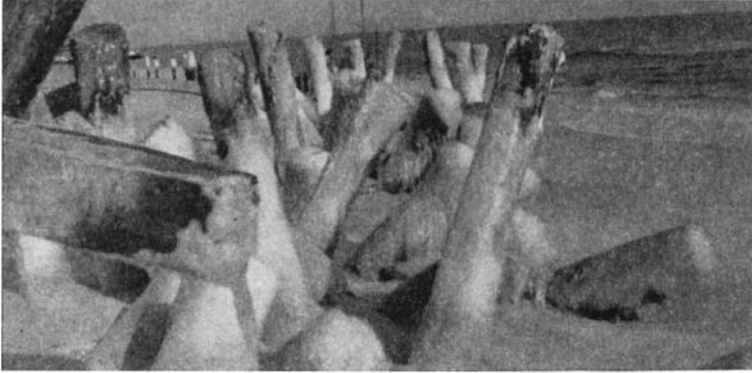
As the obsolete jetty looked after dynamite had cut pilings off below the surface and before being dragged from the sand by a horse team
