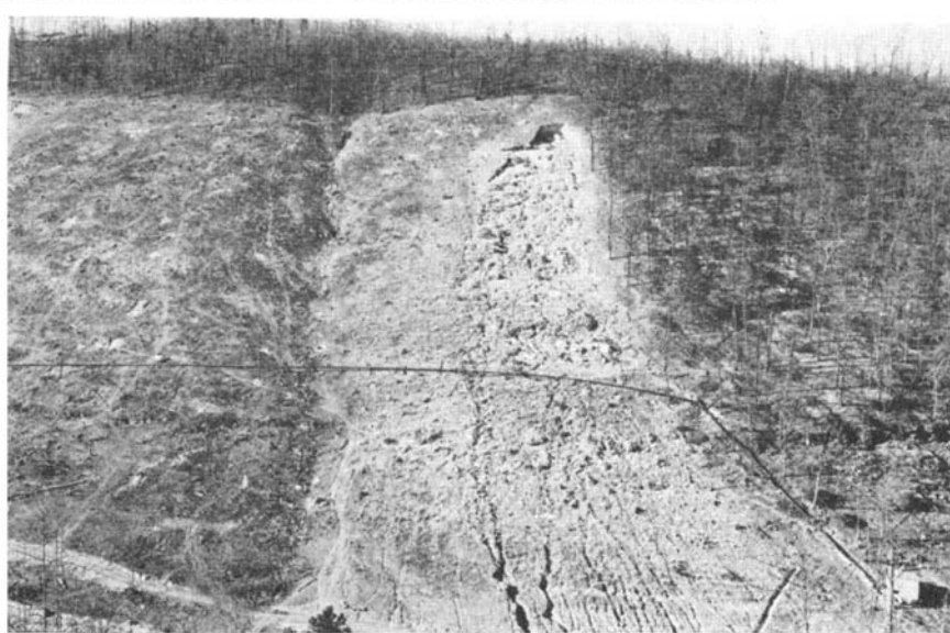
(Continued from left) the hillside to be caught in a series of check dams. The material collected is being used as a fill for a coffer dam on the west side of the dam proper. Above: General view of the quarry after sluicing operations started
