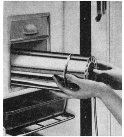
Right: The parts of the new ice-cream freezer. Motor is in end of tube. Above: Placing the freezer in the automatic home refrigerator
