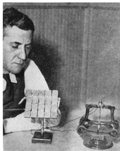
A motor that derives power from sunlight; and its light-sensitive cells
