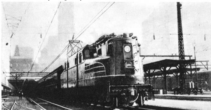
One of the new giant electric locomotives described above
