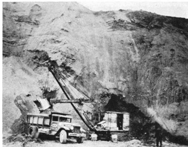
Huge hills of volcanic ash and sand present another problem. 16,000,000 cubic yards of material will be moved
