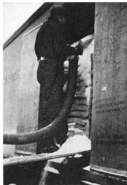
Left: The "ice-slinger" mounted on a truck, pulverizing blocks of ice. Above: The delivery hose "slings" snow ice into a refrigerator car
