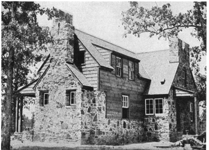
A subsistence homesteader's "castle" at Crossville, Tennessee—and it cost approximately 2000 dollars! This low cost was possible because virtually all raw material used on this project is available nearby. The homesteaders contribute labor, being paid half in cash and half as credit toward purchasing homes of their own
