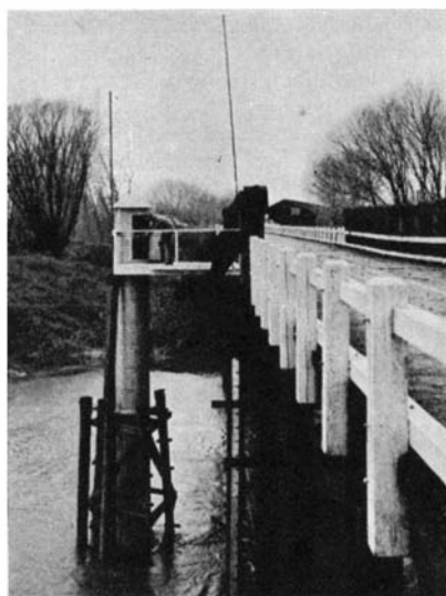
The flood warning device is in the little shelter atop the gage well
