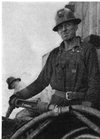
Above: Intake end of the pneumatic rivet passer, and, right, the receiving receptacle with spring buffer
