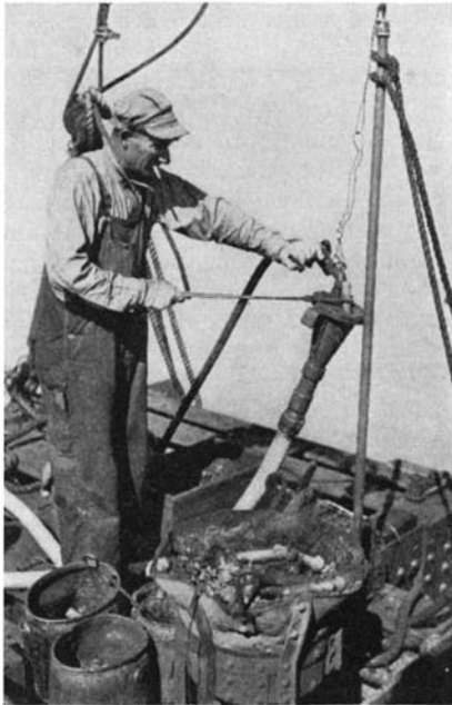
Above: Intake end of the pneumatic rivet passer, and, right, the receiving receptacle with spring buffer
