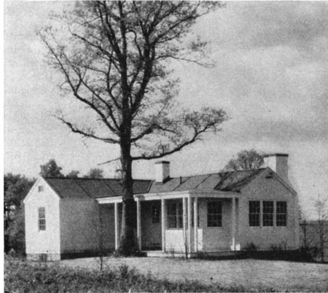
One of the houses now completed and occupied in the Experimental Community at the Reedsville, West Virginia project
