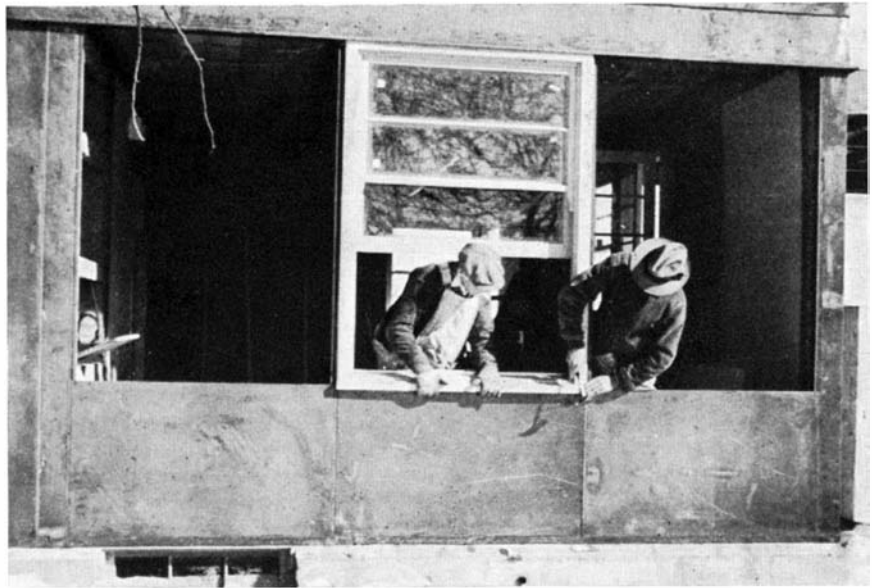
A minimum number of studs and other framing pieces are required in this pre-fabricated modern steel house. Above: inserting window frames. At left: constructing the porch roof over a steel framework
