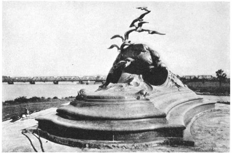
The Navy and Marine Memorial, largest aluminum monument in the world, in which many of the pieces were cast by the lost wax process
