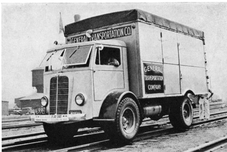
The road-rail truck during its recent trial run
