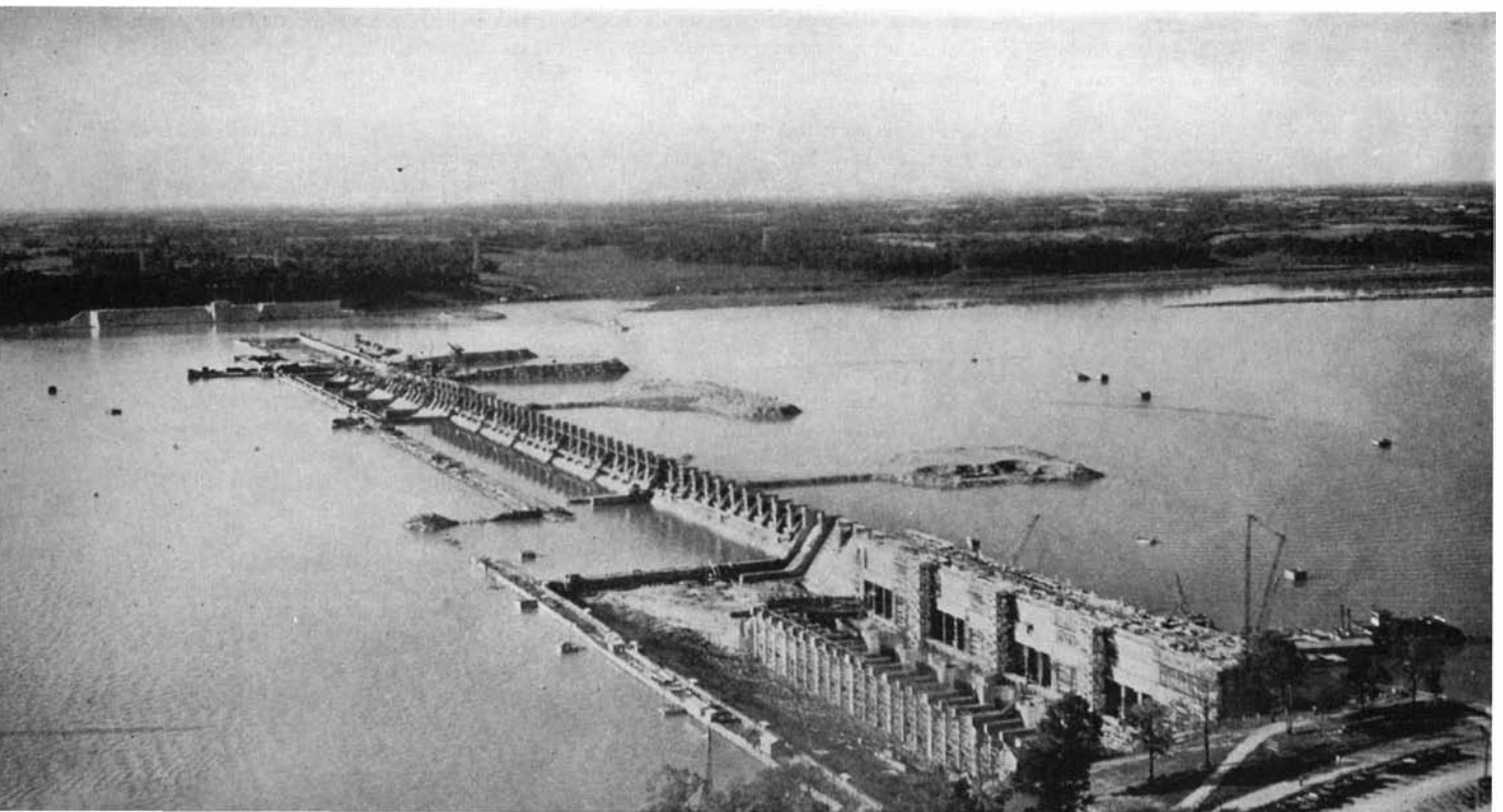
Wheeler Dam in June 1935. The navigation lock is on the opposite side of the Tennessee River
