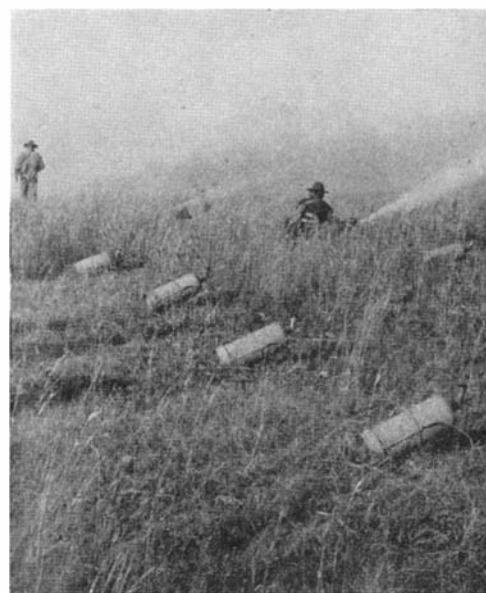
Gas cylinder attack: chlorine and
