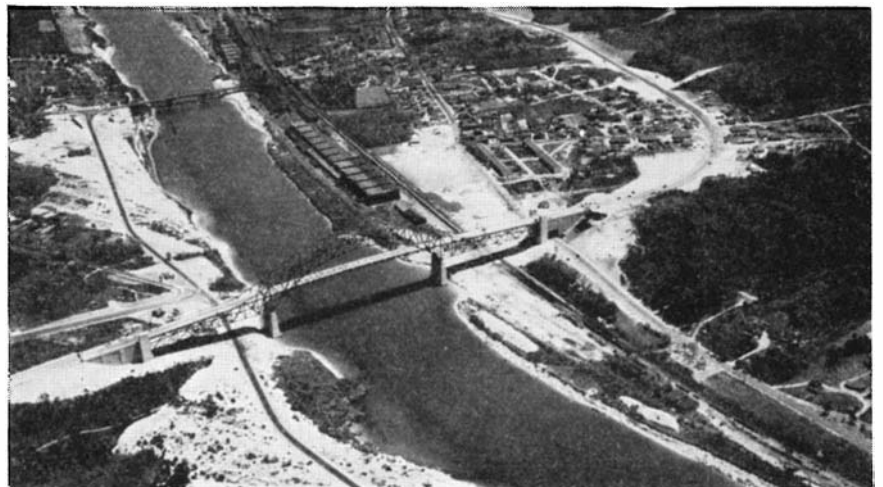
Air view of the fine new Sagamore Bridge which has a clearance of 135 feet above the waterway. Just beyond is the old one that is to be demolished very soon
