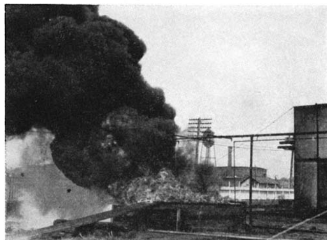
"Before and after" photographs of an oil fire that was controlled with water sprays
