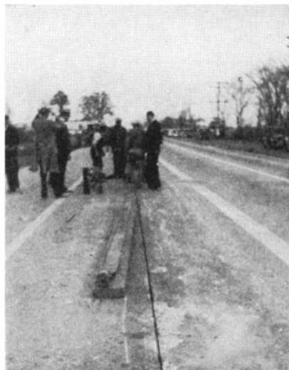
Ready to insert the three-inch hose in the unusual highway-moving system described in these columns
