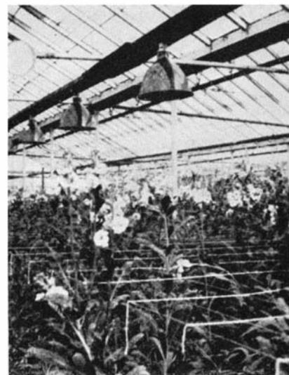
High-wattage lamps permanently located near roof of the greenhouse
