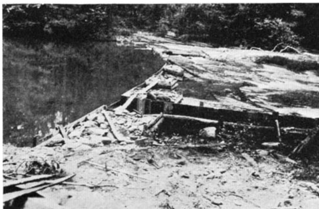
The low dam and part of the flume that leads down stream to the site of the undershot water wheel and power plant
