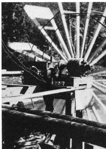
Close-up of generator and motor-car parts of homemade power plant
