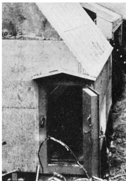
A new type of greenhouse with the walls built of insulating material
