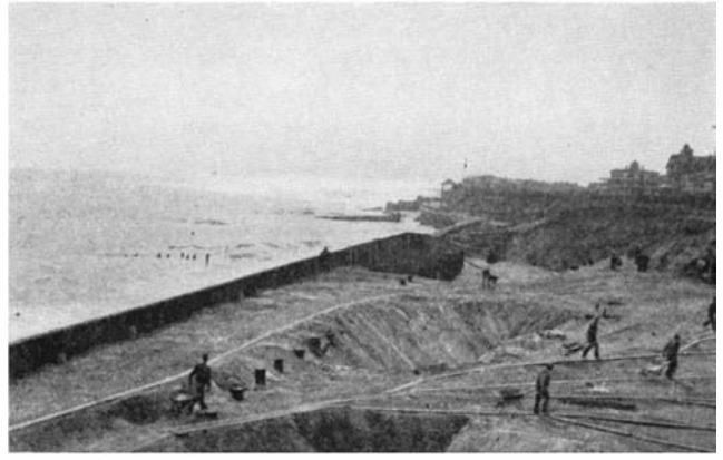
By contrast—a fine new sheet piling bulkhead at Deal Beach supported by timber bracing and wide back-fill
