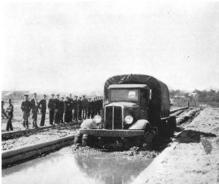
Proving that a depth of 18 inches of mud is no fit highway for a truck. This powerful military truck stuck tight in the mud course at that depth
