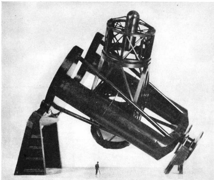
A simple little wooden model, incomplete in several respects, of the mounting for the 200-inch mirror. It is being studied by the Engineering Committee
