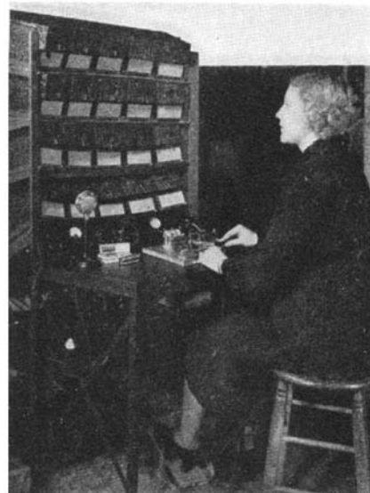
Above: An operator at the board of the new visual reed tuner for musical instruments. Left: Close-up of one of the lighted indicator panels
