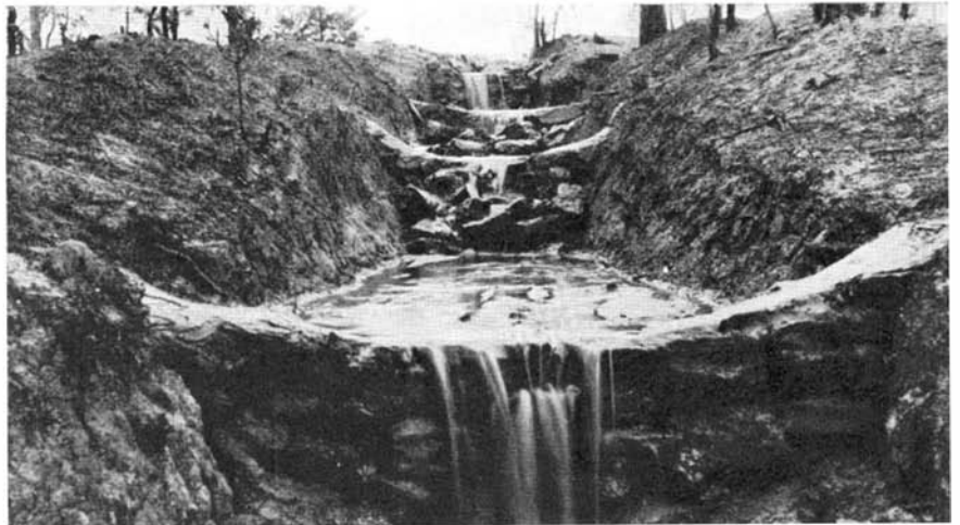
Above: A series of cemented rock dams is necessary in some cases where the gradient is steep and the erosion is fast
