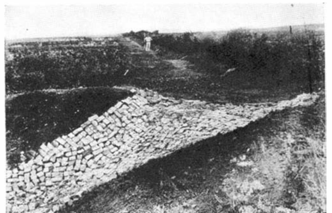
Below: An apron of loose, heavy stones, overlaid with hog wire to hold the stones in place, prevents the scouring of a hillside where run-off of storm water is heavy
