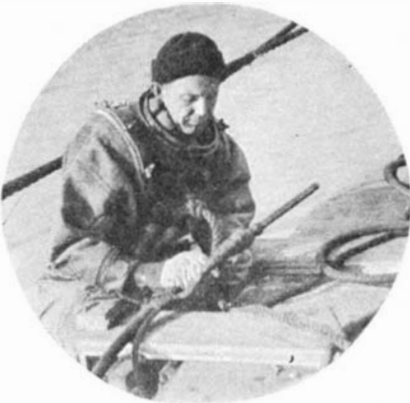
Diver, with cutting torch, before donning helmet to work submerged
