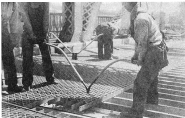
Squeeze-ripping units of the new grate decking for bridges; and a finished deck
