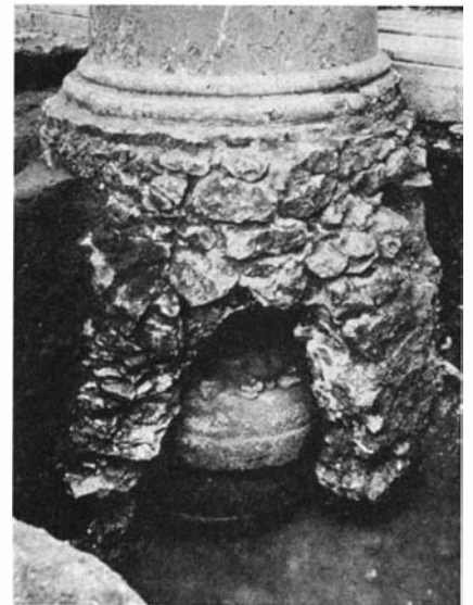
Figure 3: "Dug down outside and cut a hole in the foundations"
