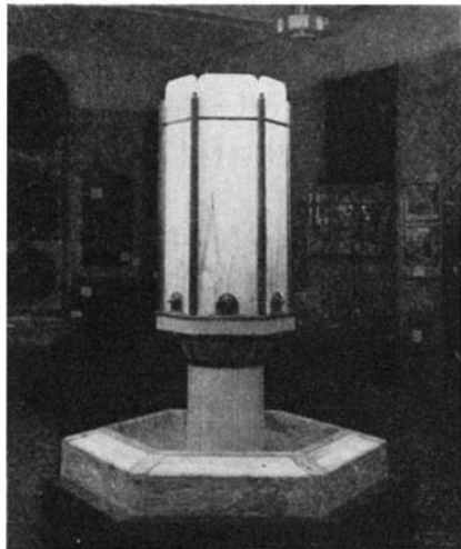
Marble panels lighted from within
