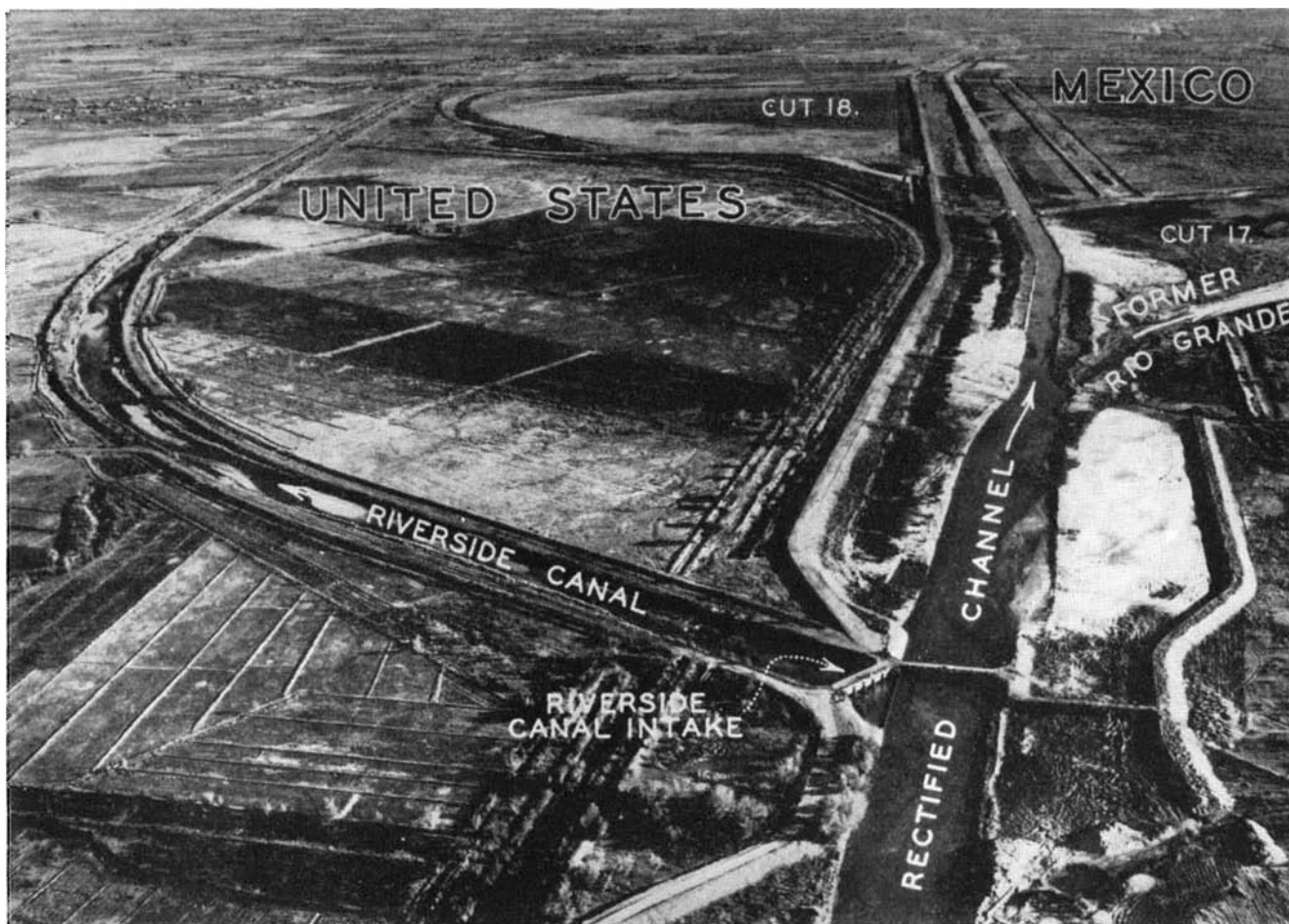
One of the principal canal intakes from the new channel for irrigation in the El Paso Valley
