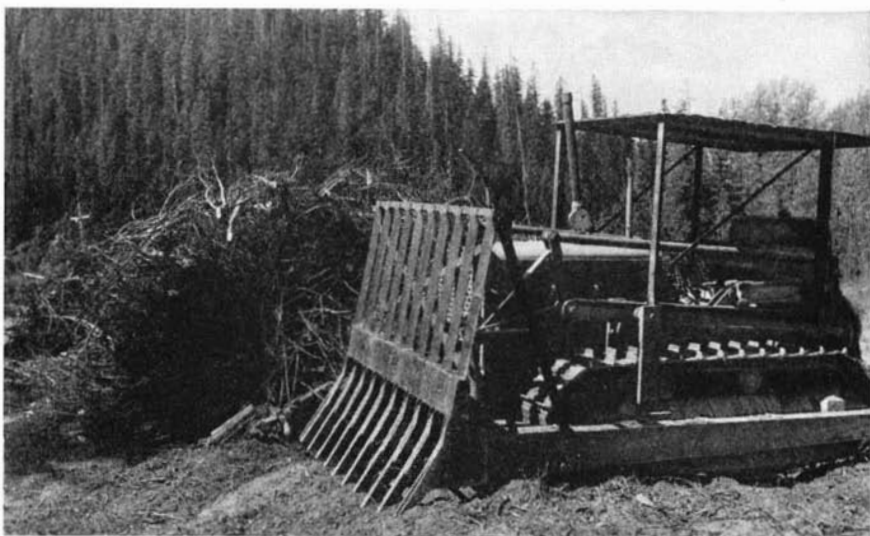
The tractor and bulldozer with special brush-removing blade
