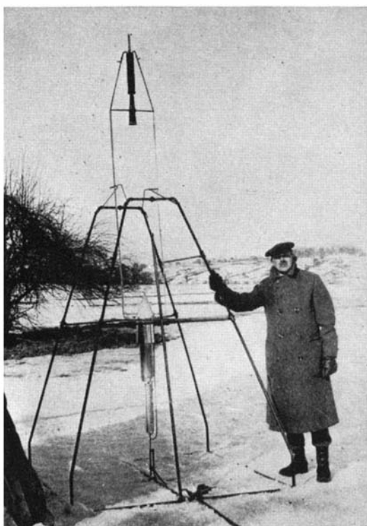
Figure 1: The first liquid oxygen-gasoline rocket, in the frame from which it was fired
