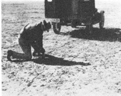
Figure 10: Cable being unwound between the tower and the shelter
