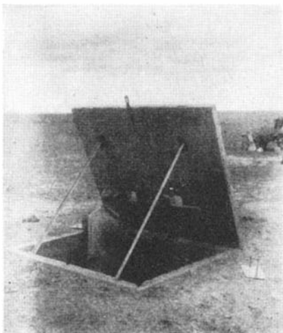
Figure 14: Concrete dugout permitting observation at close range
