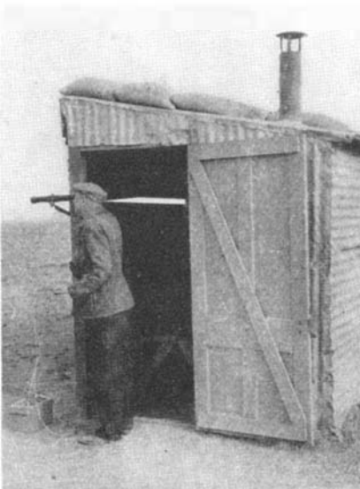
Figure 11: Control keys being operated at shelter. Note sand bags
