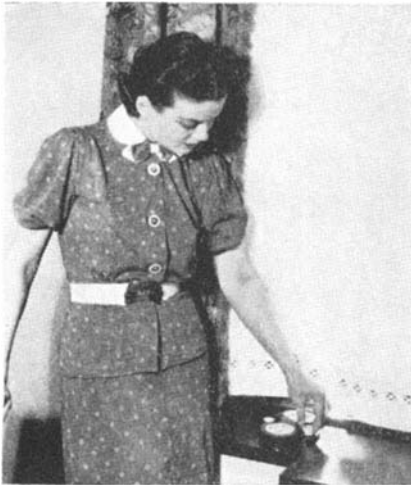
One of the individual room controls in a hotel air-conditioning system
