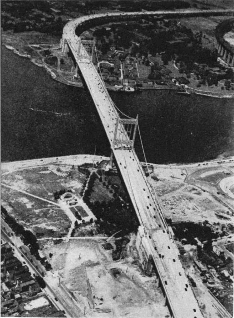
The suspension span over Hell Gate, looking from Queens. The main span is 1380 feet long, the side spans 705 feet. Vertical clearance over the river is 135 feet. Width over all is 113 feet, and the towers are 315 feet high. The span is stiffened against wind by trusses 20 feet in depth and a system of bracing below the roadway. The roadway itself will safely accommodate eight lanes of motor car traffic
