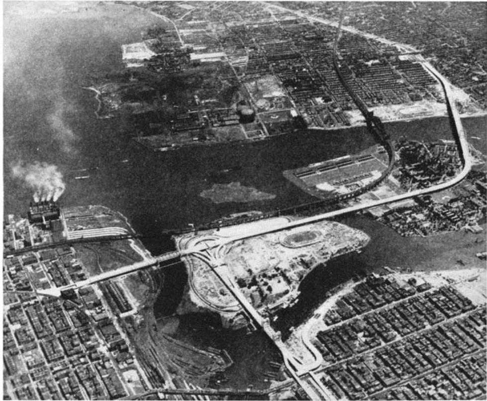
Aerial view of the Triborough Bridge, showing the completed project and some of the approach highways, which, in themselves, constitute a remarkable system for speeding up and by-passing traffic around congested thoroughfares. The traffic divider on Randall's Island (see also our front cover) eliminates all grade crossings, enables traffic to go its way without interference, and permits the collection of tolls with a minimum loss of time
