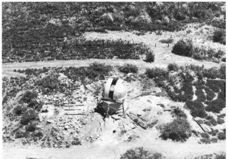
Dome for the (relatively) small 18-inch Schmidt telescope camera, which is being constructed at about 1000 feet distance from the main observatory dome
