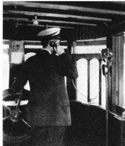
Control equipment for the marine radio telephone service is within easy reach of the pilot of the tug
