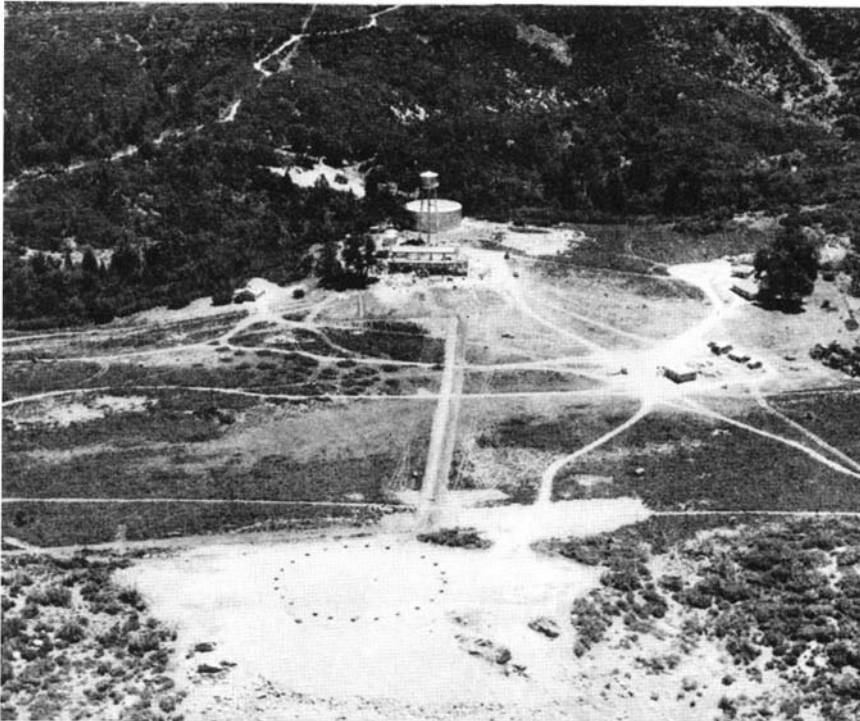
The observatory site, looking about north-east. In the foreground are holes for footings for the steel columns for the dome. In the middle is a potential landing field (see front cover). Center background: power house and water tanks. Water is pumped from the canyon beyond, 500 feet lower. Right background: Officials' residences (near trees) and temporary workmen's camps
