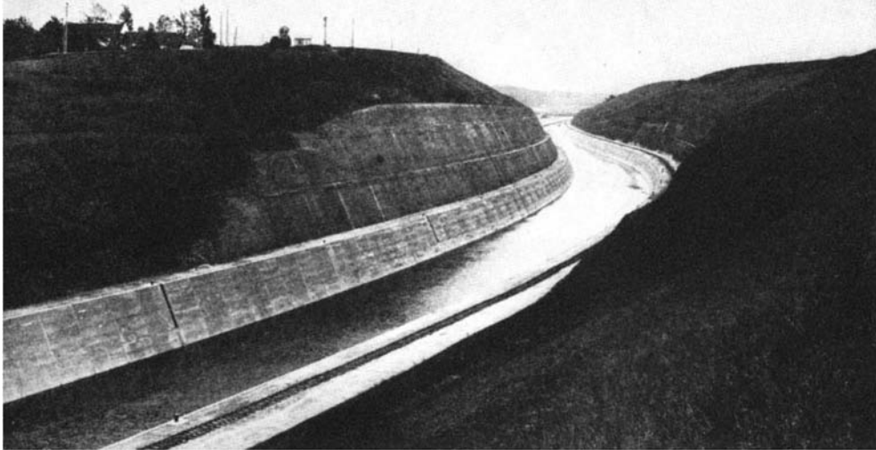
The Vroenhoven Cut, 186 feet deep, through which a large volume of canal traffic is already moving between Liège and the coal fields of the Campine Basin. Note reinforcement of banks
