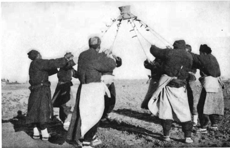
Like tossing a man in a blanket, the flapper is tossed by Chinese to compact soil. Below is the heavy flapper with eight handling ropes
