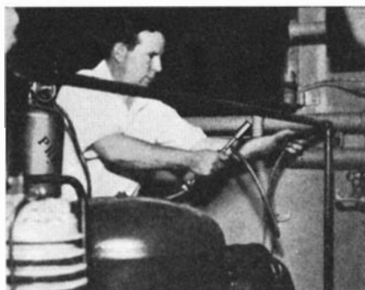
Looking for gas leaks with a flame!
