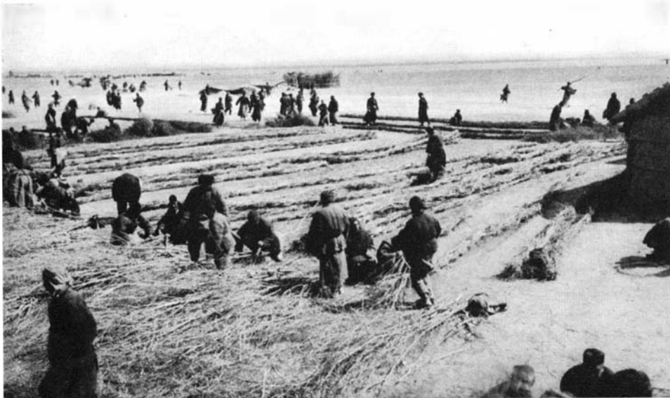
Making willow fascines in a work yard near the dike
