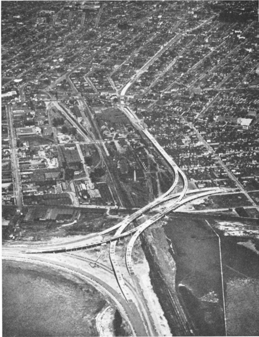
Motorists entering and leaving the Oakland end of the bridge will use this distribution structure on which there will be no right-angle crossings or left turns
