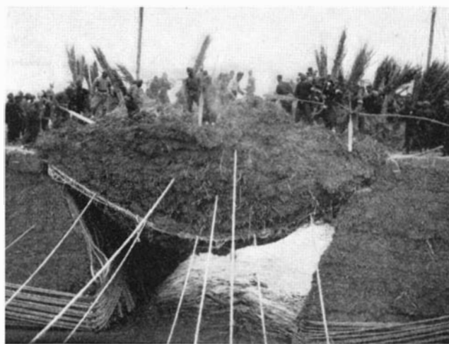
The "dragon's net" is ready for closing the secondary dike; and, at right, the kaoliang plug is being constructed thereon
