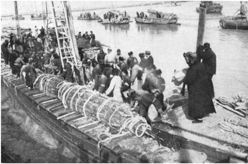
A "sausage" of stones and willow withes, ready to be dumped from a boat
