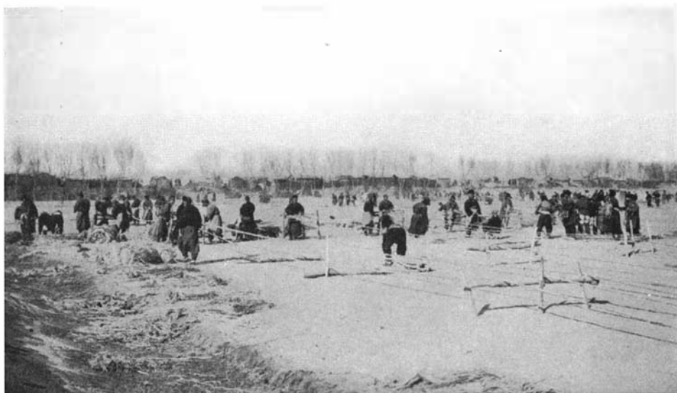
Twisting hemp into ropes by the ancient Chinese method; and, below, the ropeway near the dike job
