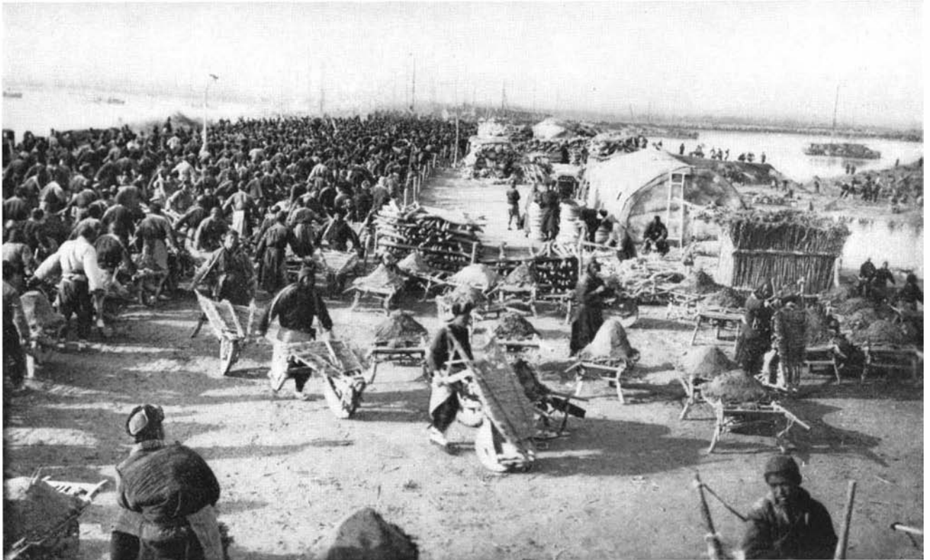
Tramping on one another's heels, perhaps, but not WPA workers; these Chinese are working hard for 10 to 15 cents per day. For half a mile back from the working face of the dike under construction, loaded wheelbarrows occupy all available space
