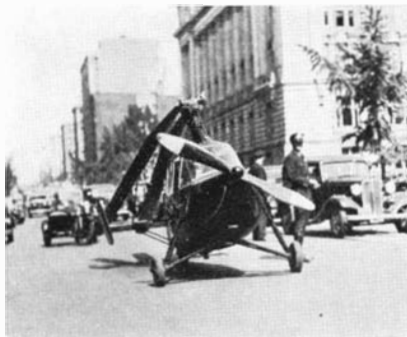
Above: The roadable Autogiro in a city street. Below: Side view of the 'giro with the two vanes folded ready to be run along any highway
