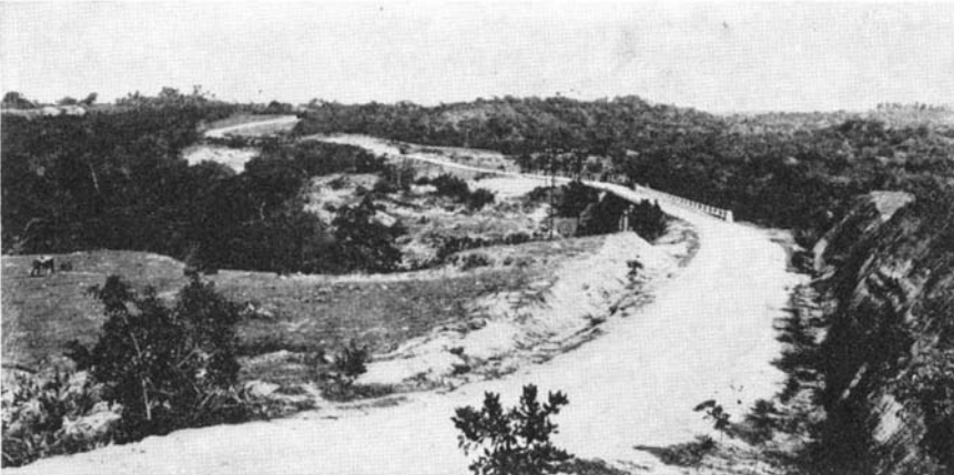
Below: A section of the Central Highway of Panama which is included in the route of the Inter-American Highway
