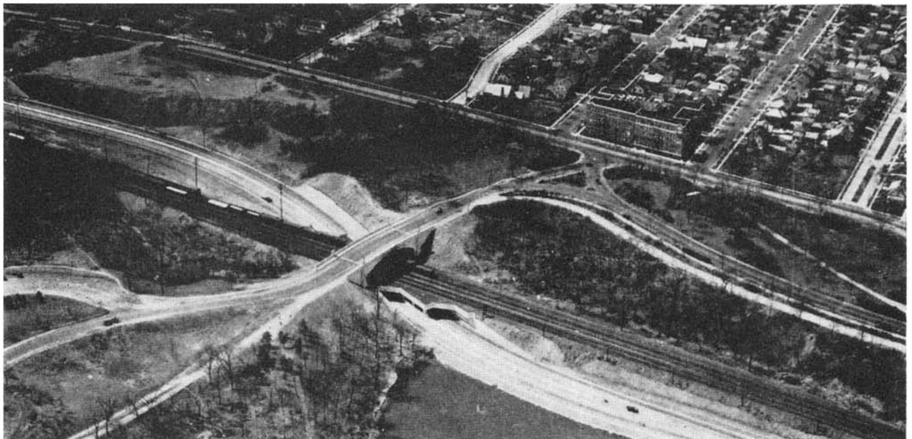
Traffic on three levels. Two separated highways with a railroad right-of-way on the center level
