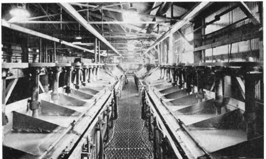
The flotation floor in one of the modern molybdenum recovery plants
