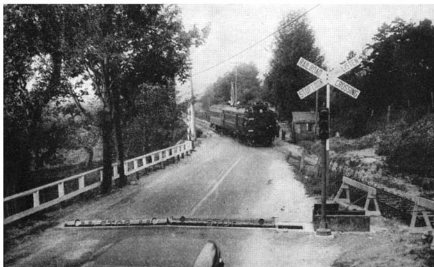
A "bump-stop" signal, automatically operated, for railroad crossings
