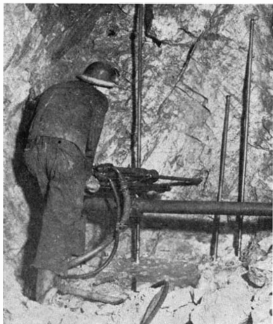
Drilling preparatory to "shooting" in one of the main headings of the huge moly mine
