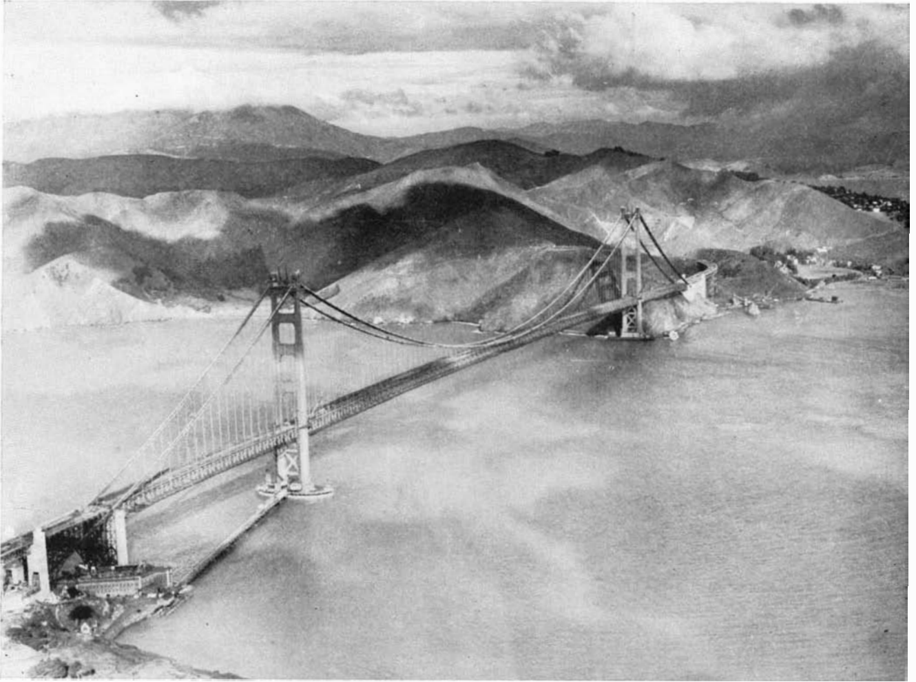
Recent air view of the Golden Gate Bridge, with Marin hills in the background and Mt. Tamalpais at upper left
