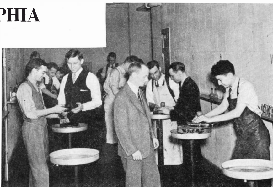
A typical Thursday night session. The photograph shows half of the available pedestals around which the concave glass mirror disks of reflecting telescopes are ground and polished by hand, using the fine abrasives shown in the bottles and shakers on the shelves
