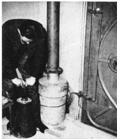
Cracks around the door of a gas-proof cellar being sealed by a soft rubber tube inflated by a pump
