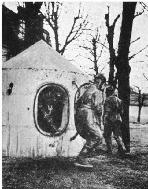
Leaving a concrete shelter, capable of housing three persons. Note the conical shell- and bomb-deflecting top of shelter
