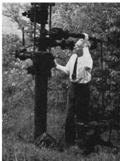
Mr. Mershon's backyard gas well
