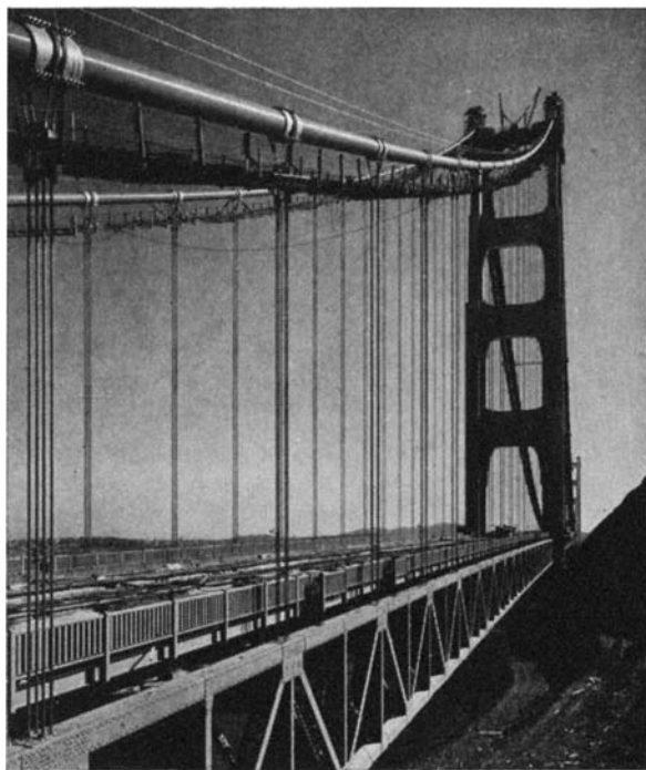
Golden Gate Bridge, where 79,792 miles of wire (in two single cables) support a span 4200 feet long
