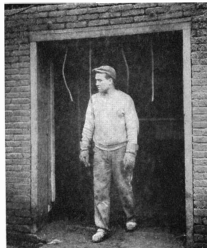
Doorways adjacent to tracks of the Bethlehem Steel Company are equipped with "cat-tails" to remind of possible approach of engines.
