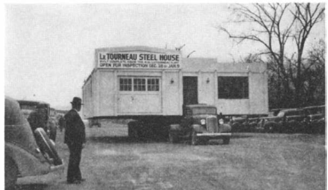
An electrically welded home, ready for occupancy, leaving the factory—and being transported by trailer
