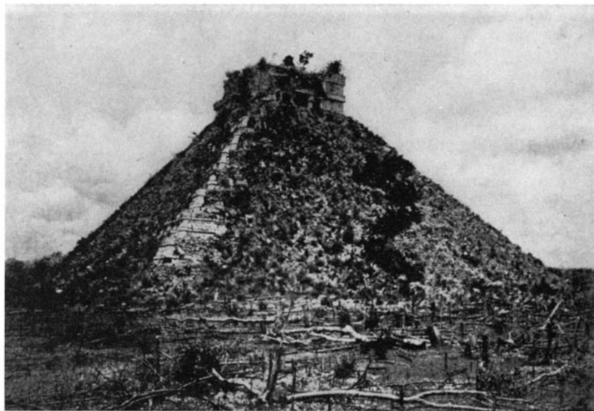
Before its restoration by the Mexican Government the old Maya pyramid was in a sadly tumbled-down outside condition. Trees grew over its damaged faces
