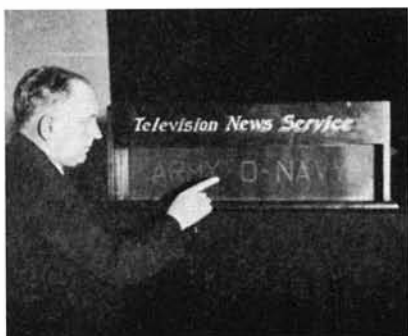
Above: Special cellophane tape being fed into the television news transmitter. Below: The shadow-box of the receiver, showing how bulletins are reproduced
