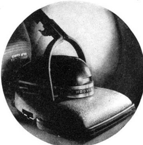
Magnesium alloy die castings plus plastics cut weight, enhance design
