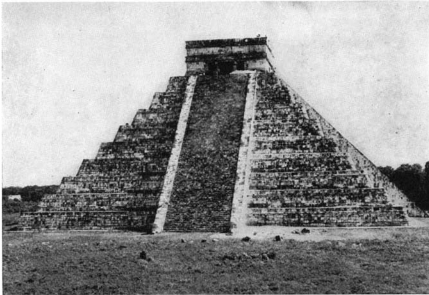
The great pyramid, 79 feet high and 197 feet wide, as now restored, showing the northern face. Stone stairways rise to the summit on each of the four faces
