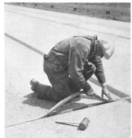
The rubber expansion joint filler for highways is pounded into place
