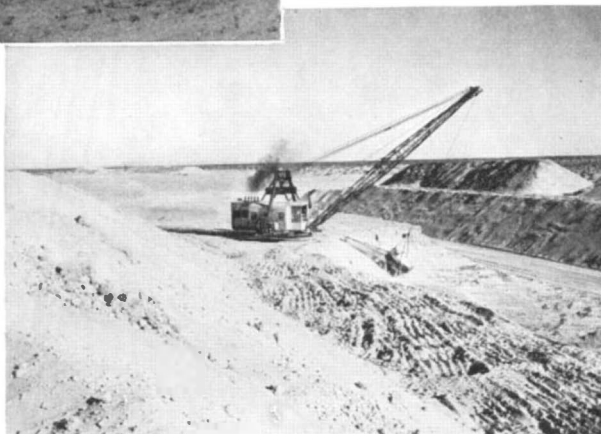
Sand and gravel in the hotter desert sections called for the use of draglines operated by powerful engines. Here, the problem of drifting sands is a big factor
