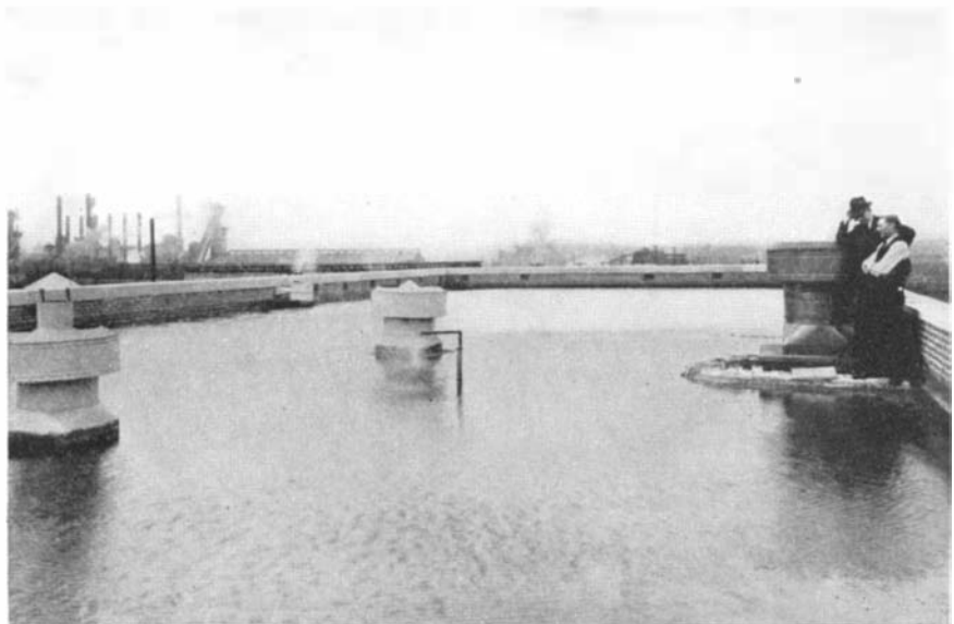
To keep buildings cool in summer and warm in winter, water insulation on roofs is the latest in air conditioning. Its usefulness is being carefully studied
