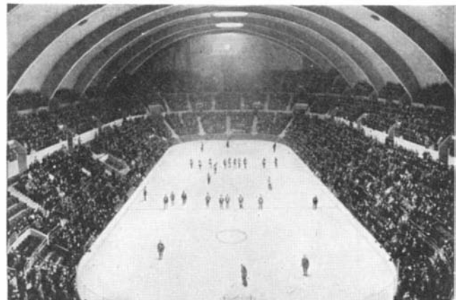
The completed 3\frac{1}{2} -inch shell roof over a first-night audience at a hockey game. No columns obstruct the view
