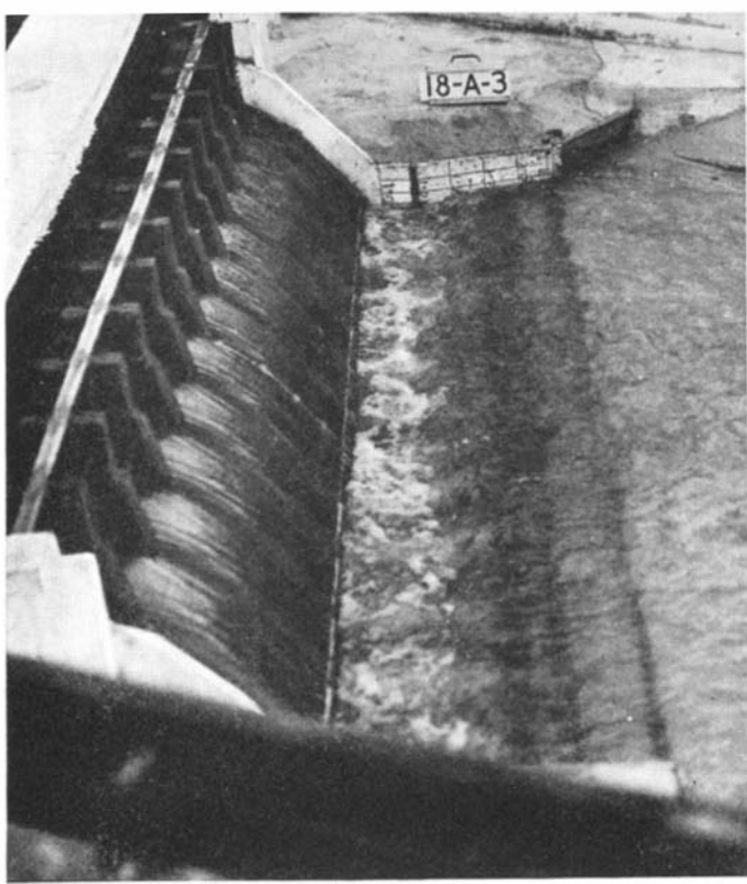
Above: Use of many dams and spillways on headwaters of the Mississippi may be one means of controlling floods. Hence the engineers study models of such dams and their spillways, a spillway model being shown here
