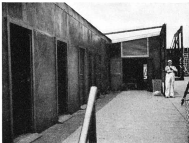
Below: The dressing rooms back-stage. The composition walls can readily be taken apart and assembled as necessary
