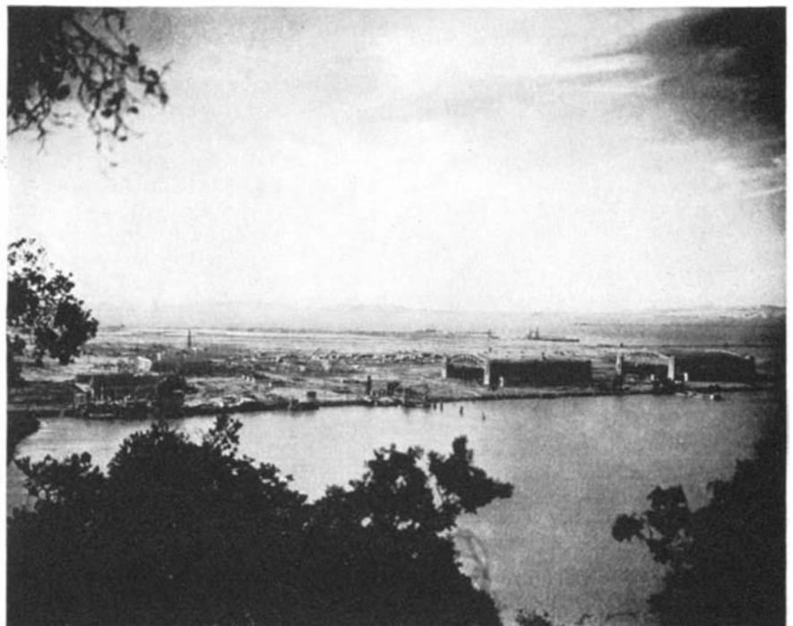
The two hangars that have been built from the roof down. See text
