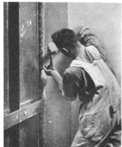
With socket wrenches, a trained crew bolts bulkheads into position
