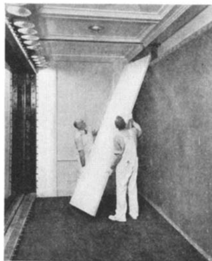
Decorative paneling, normally secured by dowels, is then taken down
