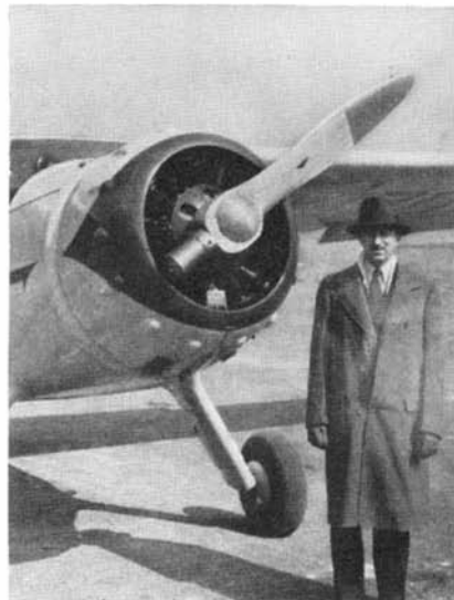
The single-blade variable-pitch propeller on a Fairchild cabin plane
