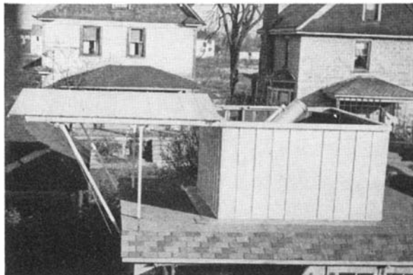
Figure 2: Mason's garage roof garden
