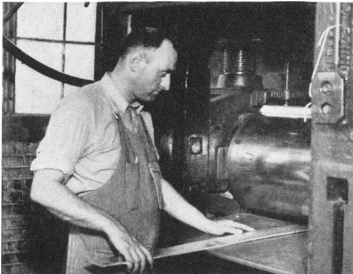
Below: No delicate jewelers' tools here—heavy machinery rolling out platinum sheet into workable strips
