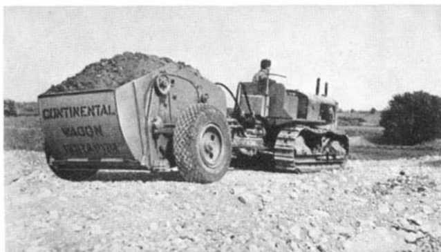
Hauling a load in the new four-yard scraper, and dumping it
